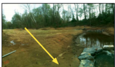
Figure 2. Project partners removed three feet of accumulated sediment and reconnected Watts Branch with its historical stream channel. Before the restoration effort, Watts Branch followed the path denoted by the yellow arrow.
